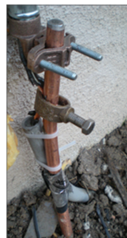
Grounding Electrode Connection
