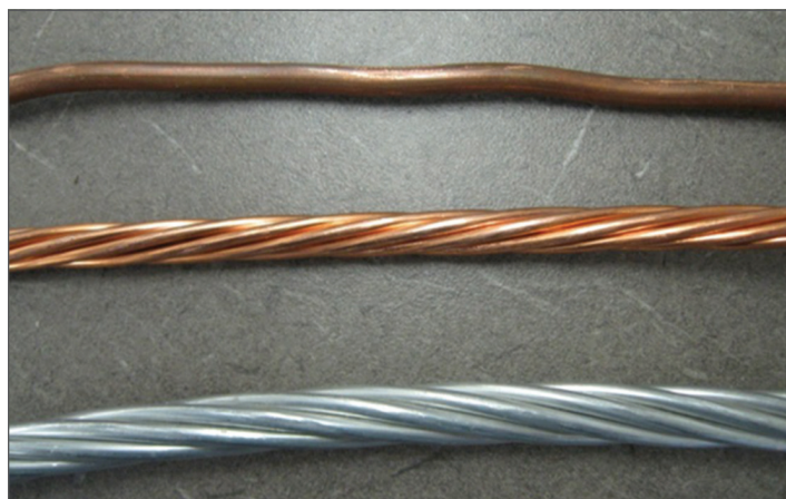
Example of Bonding Conductor
